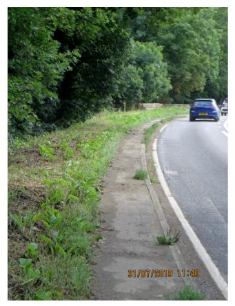
A4095 between Bladon and Hanborough Rail Station showing existing footway requiring widening and resurfacing to provide a new shared cycle footway
