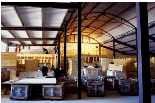
The adjoining warehouse delivers vast volumes of warm air from the roof space
