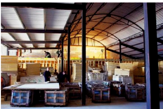
The adjoining warehouse delivers vast volumes of warm air from the roof space
